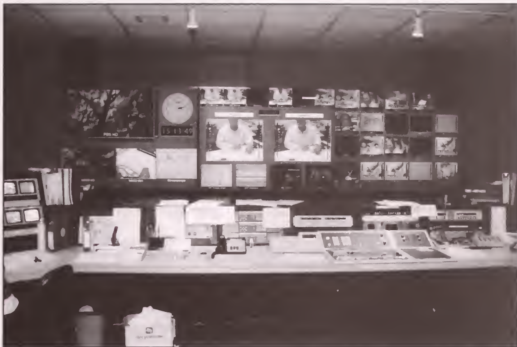
The master control room of Bridges TV in Buffalo, NY.
