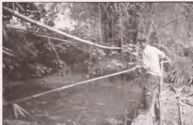
A community member unclogging pipes from one of the natural water sources on the finca
